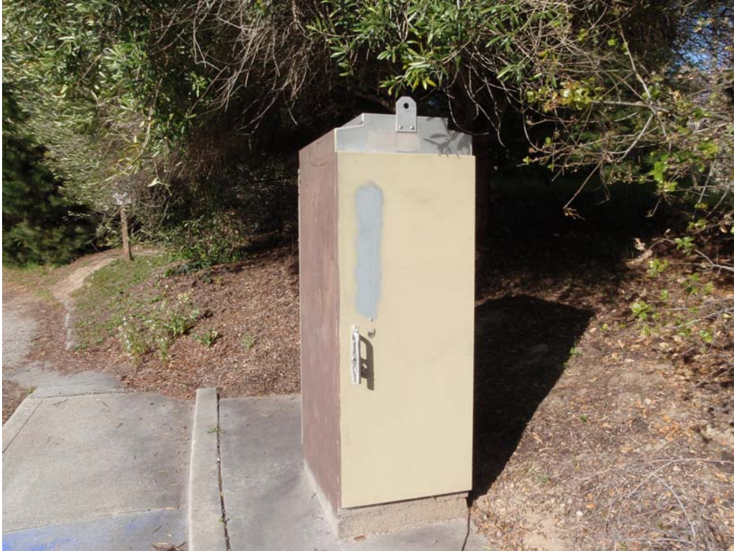
NW corner of intersection (Looking West)
