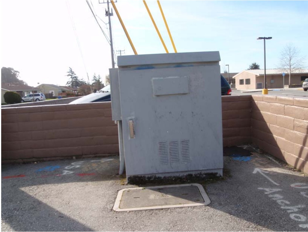
SW corner of intersection (Looking South)
