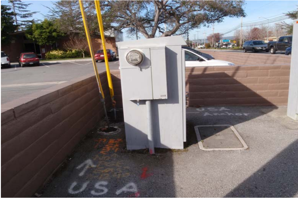
SW corner of intersection (Looking West)
