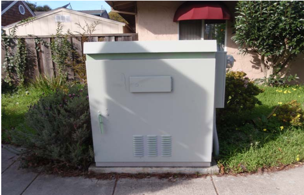
SW corner of intersection (Looking West)
