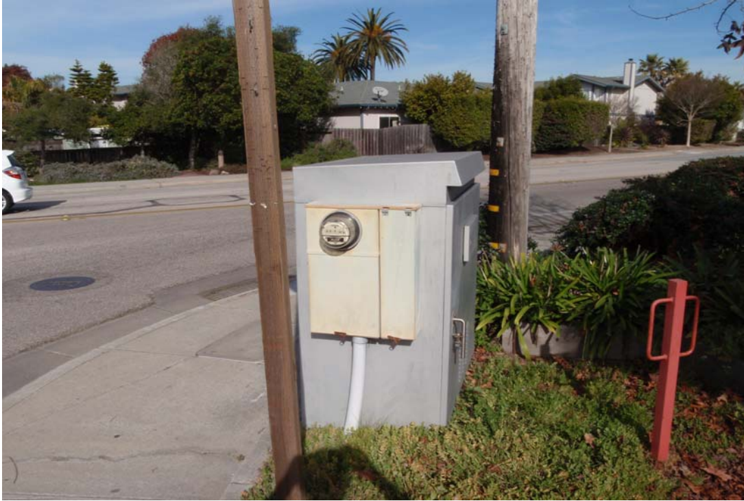
NE corner of intersection (Looking North)
