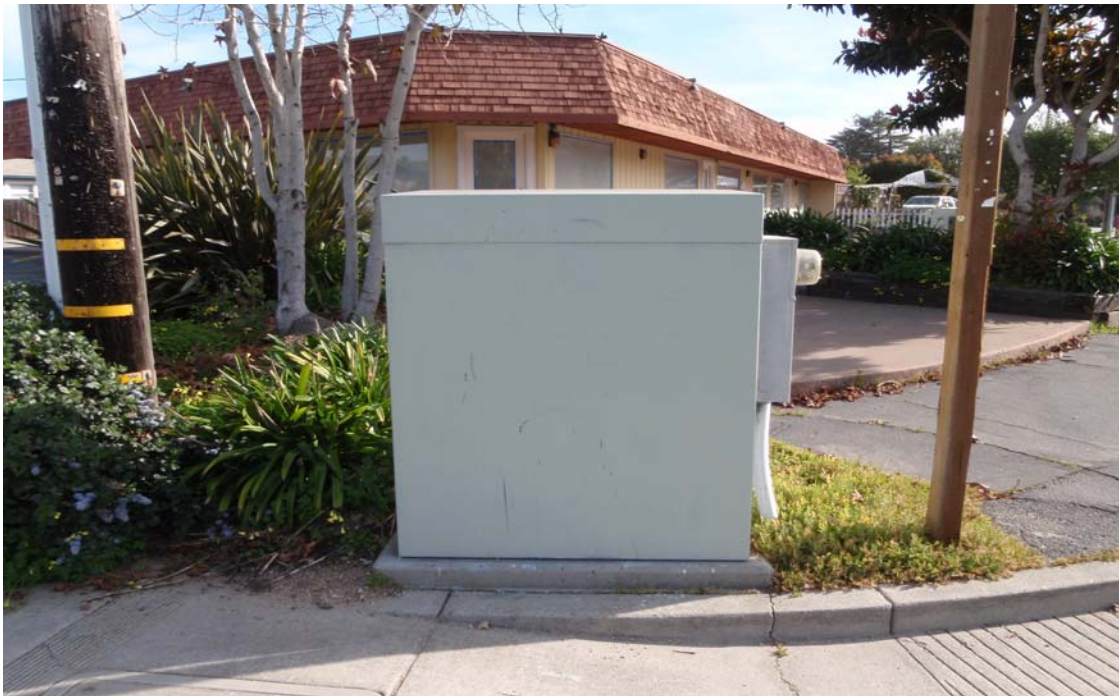
NE corner of intersection (Looking East)
