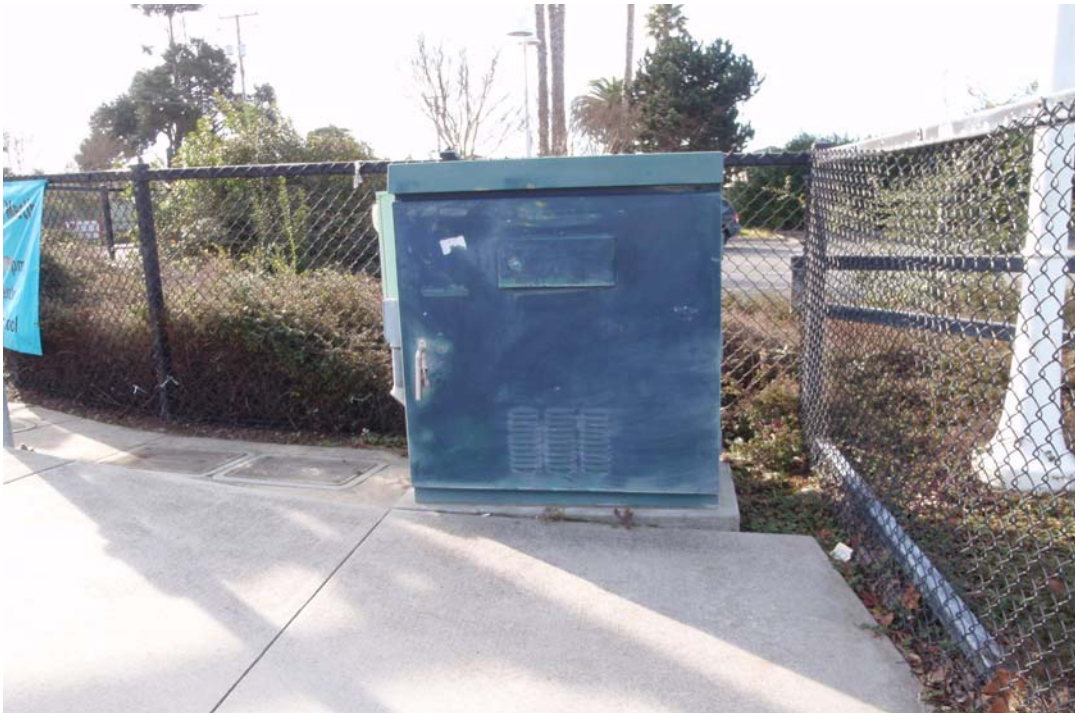
SW corner of intersection (Looking South)
