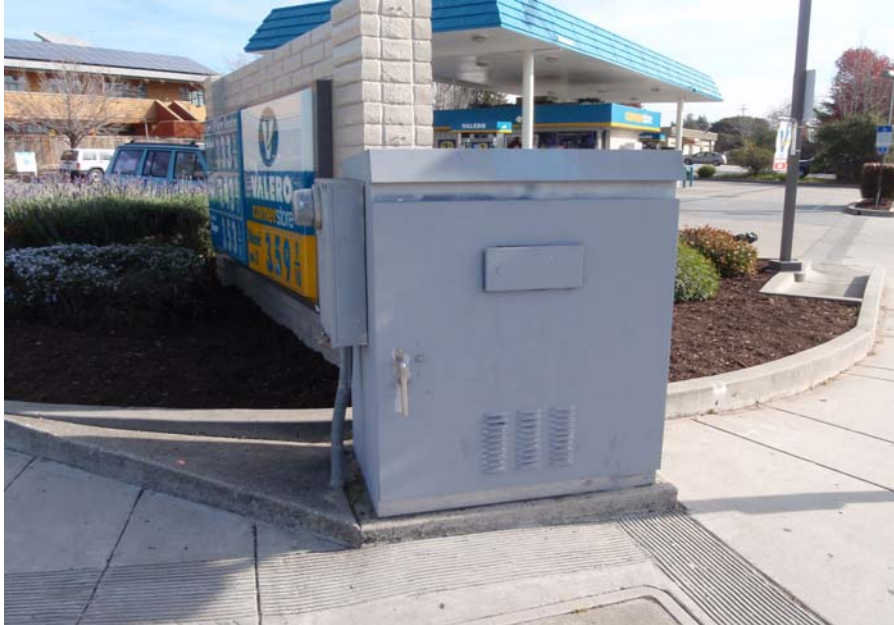
NE corner of intersection (Looking North)
