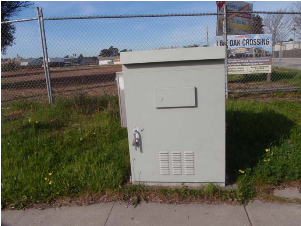
SW corner of intersection (Looking West)
