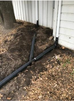
Rain gutter enhancements in Progress
